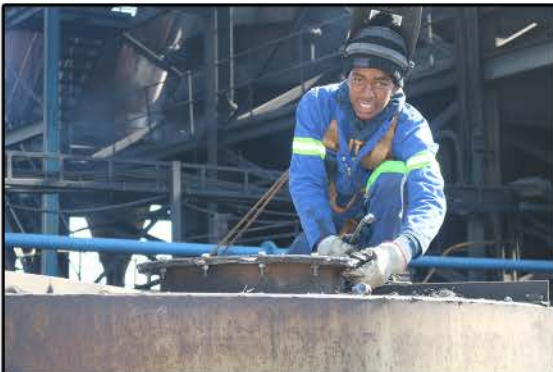
Themba Guma (Boilermaker apprentice) working at the plant.
